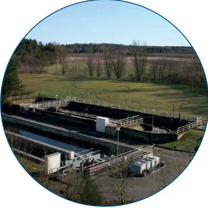
Fig. 1: Oxidation ditch with volume of 1,400 m<sup>3</sup>
